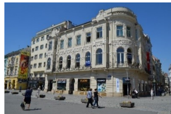
Obr.32: Budova v dobrém stavu
